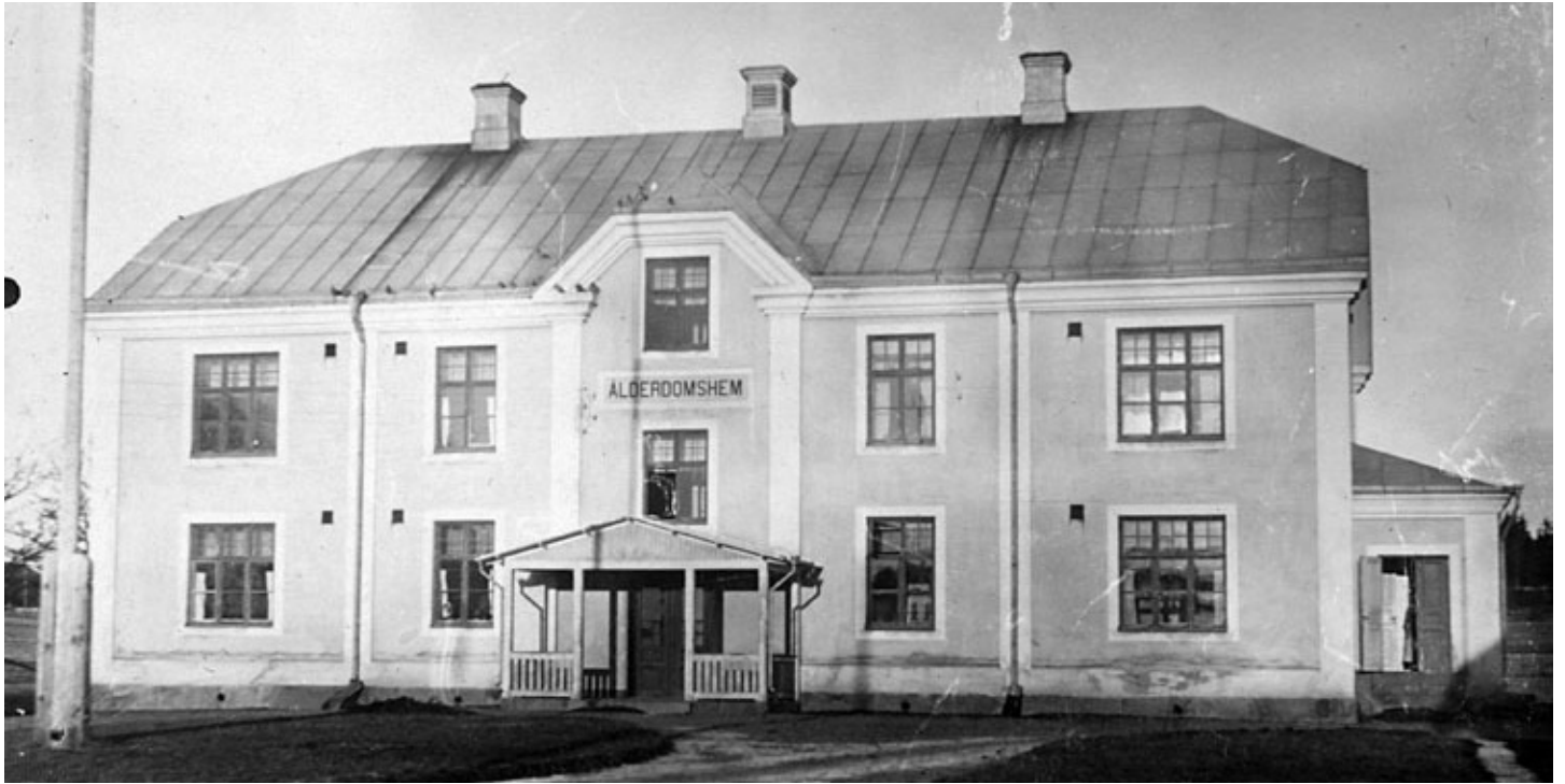
Gunnerudsgården (Residence Gunnerud) when it was a retirement home - Ö Emtervik hembygdsfören's picture archive, retrieved 210322
